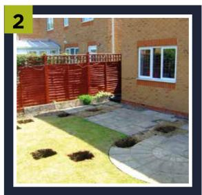
Install the concrete pads as per the pad plan supplied. Note the lack of mess and disruption!
